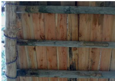
We cut and stripped trees of 8-10cm diameter and lashed them on as railings about 1.2m above the platform. To these we fastened old climbing rope to create a temporary side to the treehouse (and stop people falling off!)
