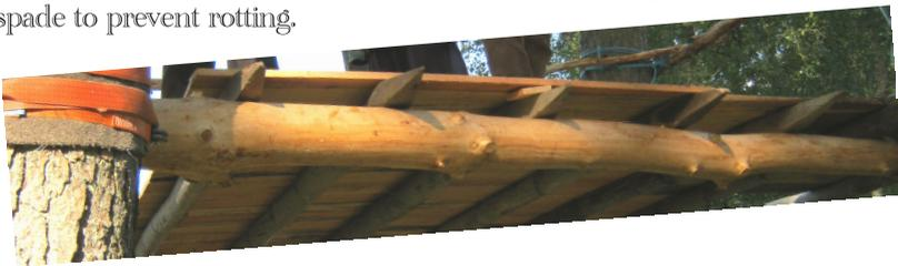
For cross beams we re-cycled old (but decent nick) fence posts, 10cm in diameter which we placed about 36cm apart. These we then nailed to the support beams. Second grade planks made the floor.
